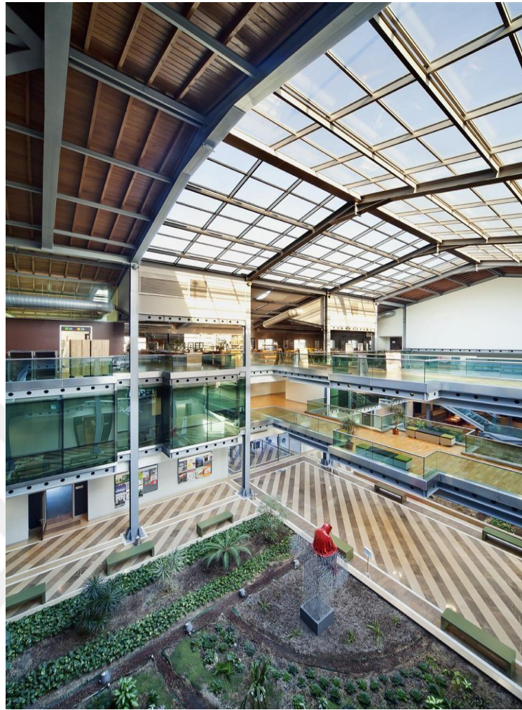
Figure 3.6 Central courtyard at block D, sourceKhas.edu.tr
